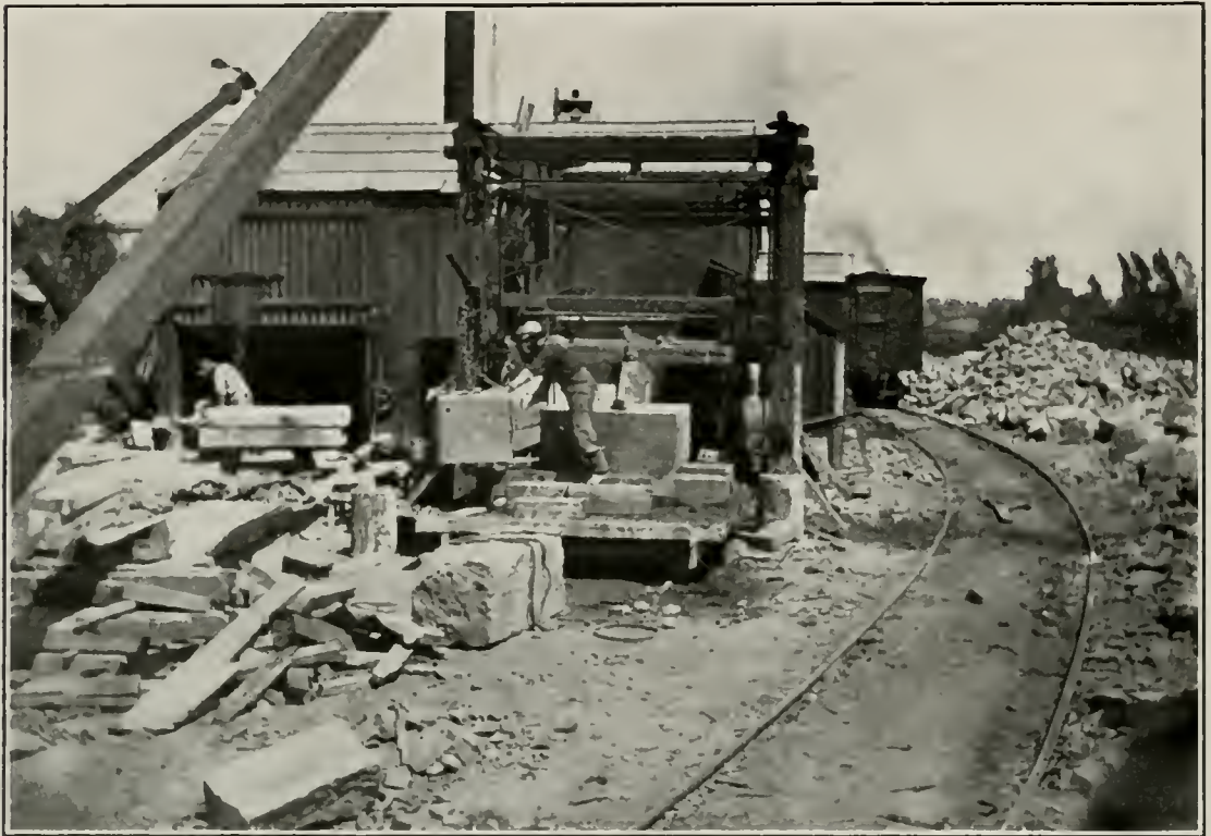
ILL. No. 12. STONE-SAWING MACHINE. BLY BROS. STONE COMPANY, LOS ANGELES.
