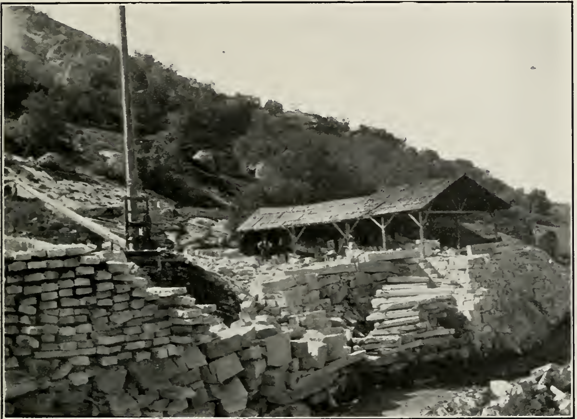
ILL. No. 21. SHED AND YARD AT ROCKY POINT GRANITE QUARRY. TULARE COUNTY.
