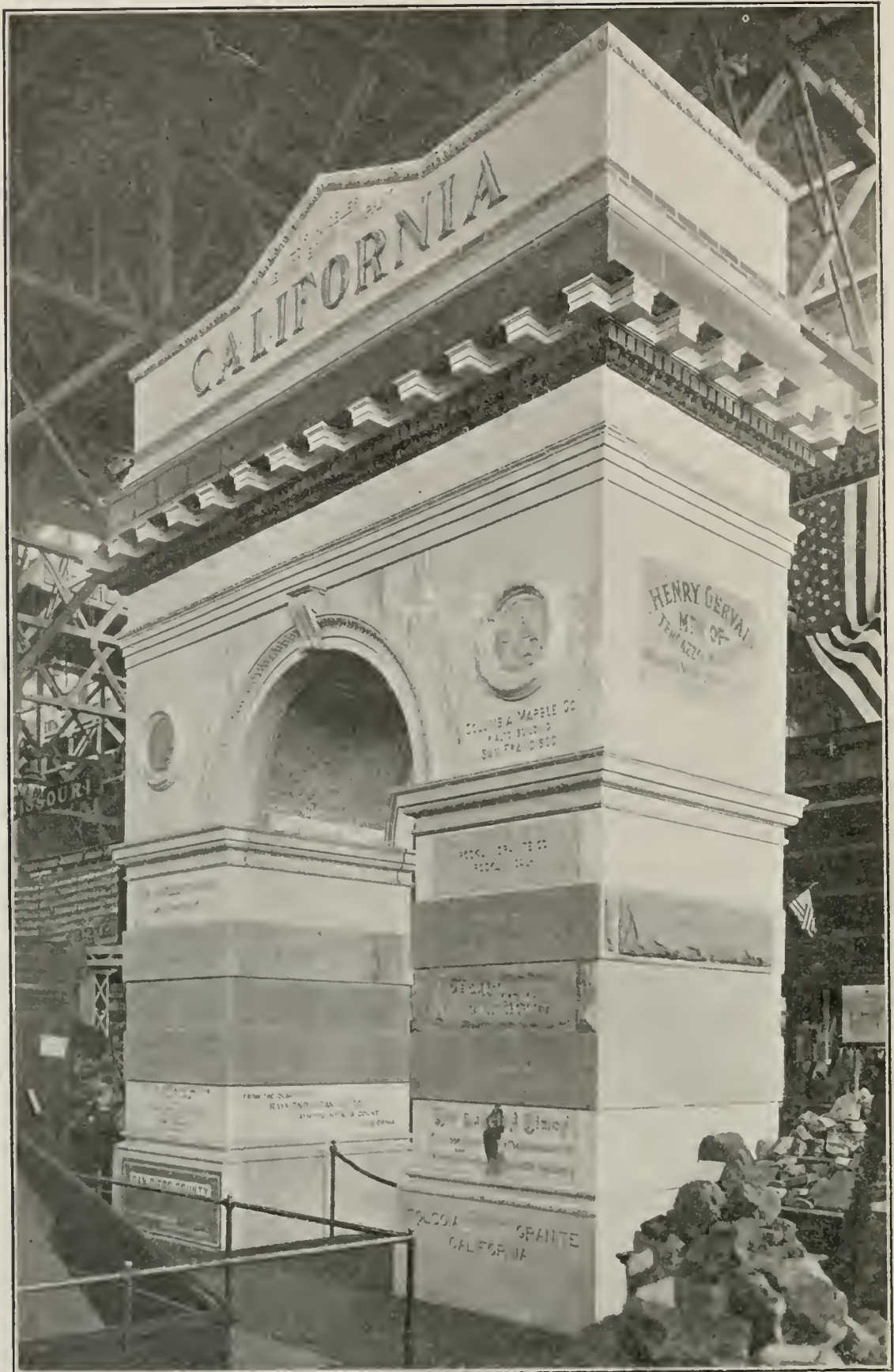
ILL No. 1. COMPOSITE ARCH, CONSTRUCTED OF CALIFORNIA GRANITE, SANDSTONE, MARBLE, TERRA COTTA, SLATE, TILING, PRESSED AND GLAZED BRICK, AT THE ST. LOUIS EXPOSITION, UNDER THE DIRECTION OF LEWIS E. AUBURY, STATE MINERALOGIST.
