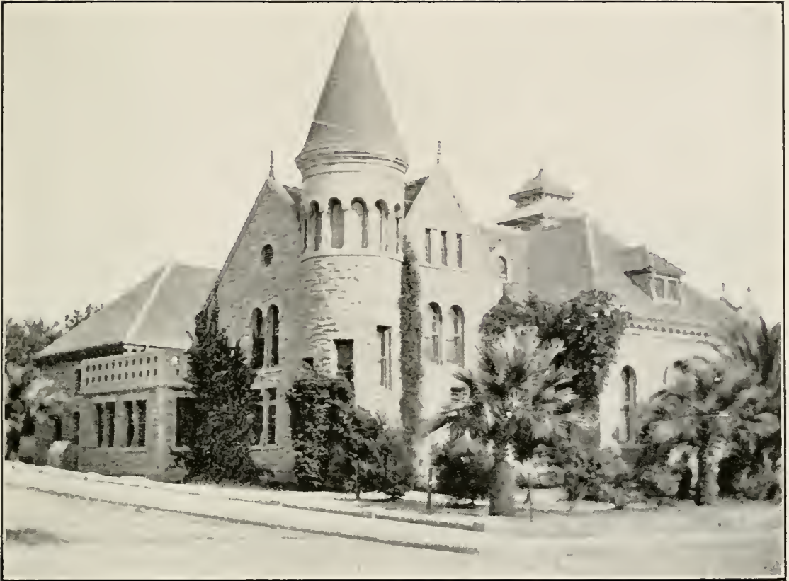
ILL. No. 58. PUBLIC LIBRARY BUILDING, PASADENA, LOS ANGELES COUNTY. Constructed of Nile-green sandstone, and trimmed with red sandstone from Kern County.
