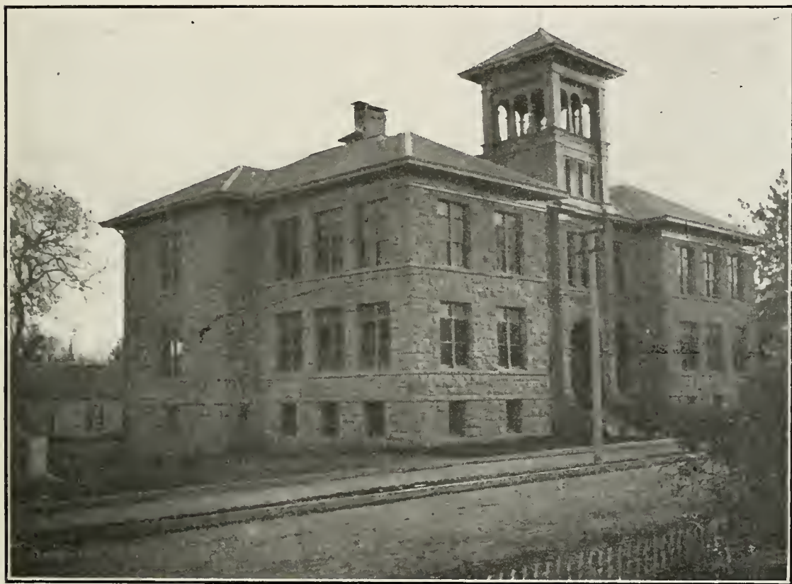
ILL. No. 71. ST. HELENA PUBLIC SCHOOL. Constructed of Trachytic Tuff from Moffat Quarry, near St. Helena Napa County.
