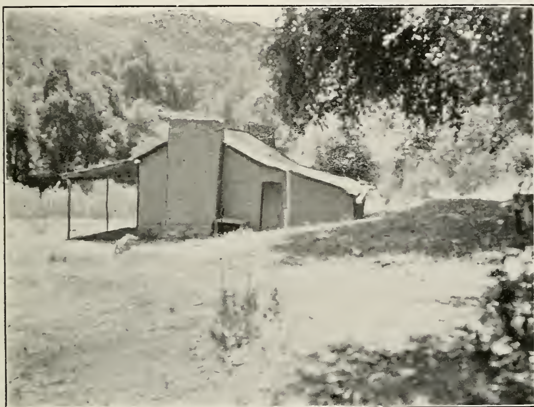
ILL. No. 104. ADOBE HOUSE, SHOWING USE OF ADOBE BRICKS. SAN BERNARDINO COUNTY.
