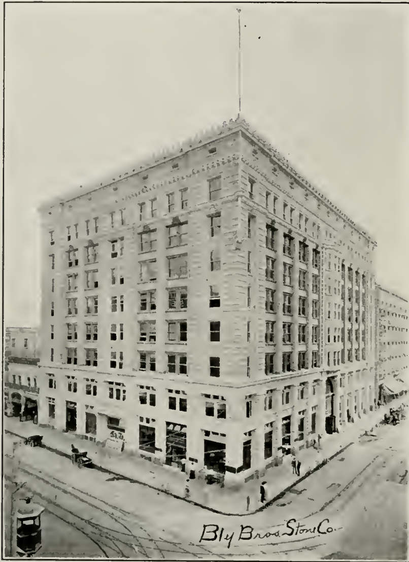
ILL. No 16. H. W. HELLMAN BUILDING, LOS ANGELES. FIRST TWO STORIES CONSTRUCTED OF RIVERSIDE GRANITE.
