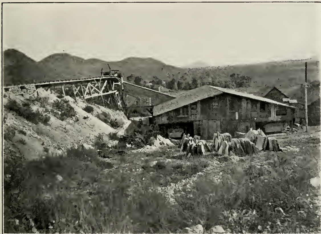
ILL. No. 39. MARBLE MILL AND YARD, COLTON, SAN BERNARDINO COUNTY.
