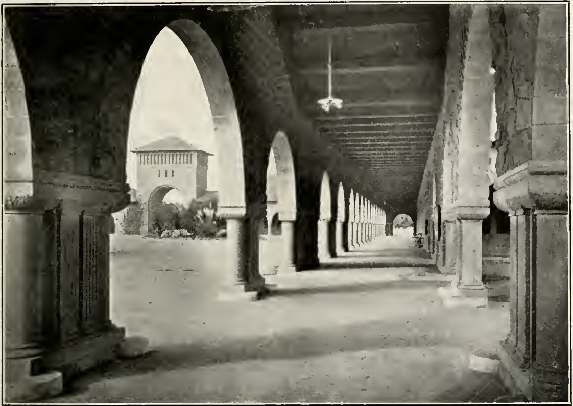
ILL. No. 48. VIEW OF ARCHES OF INNER QUADRANGLE, STANFORD UNIVERSITY. BUILT OF SANDSTONE FROM GOODRICH QUARRIES, SANTA CLARA COUNTY.
