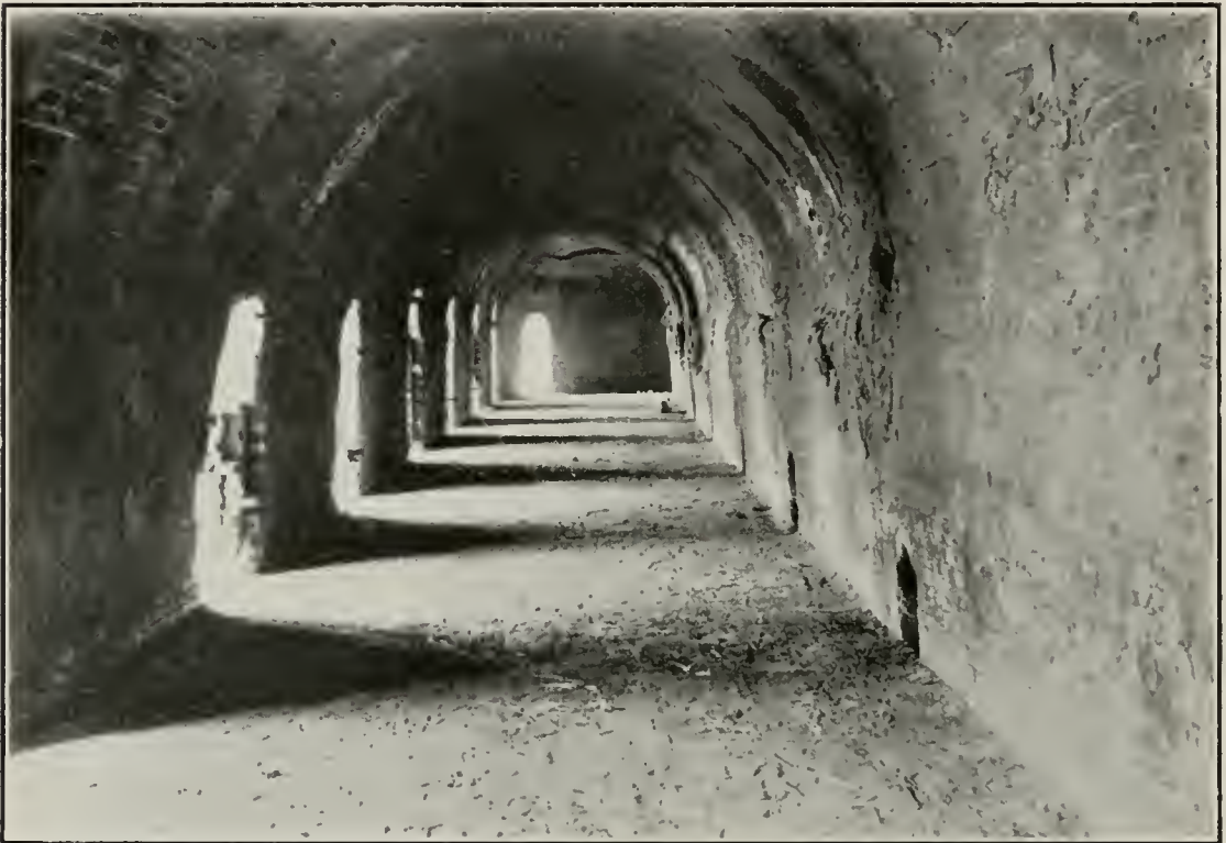
ILL. No. 111. INTERIOR OF A CONTINUOUS BRICK KILN (HOFFMAN TYPE).
