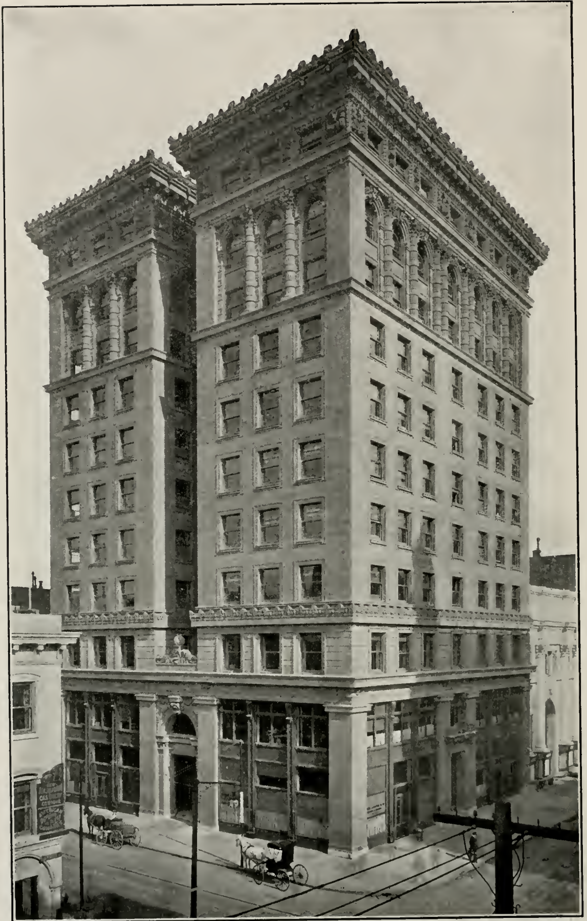
ILL. No 50. KOHL BUILDING, CORNER OF CALIFORNIA AND MONTGOMERY STREETS, SAN FRANCISCO. BUILT OF COLUSA SANDSTONE.
