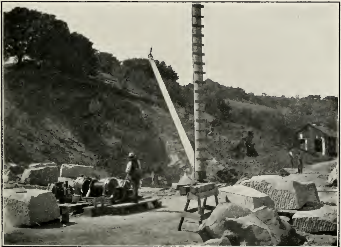
ILL. No. 55. FRANKLYN SANDSTONE QUARRY, CONTRA COSTA COUNTY. Wilson-Lyon Construction Company.
