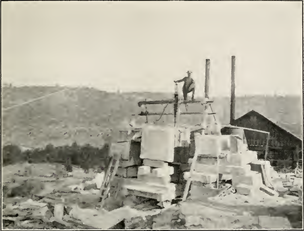
ILL. No. 2. RAYMOND GRANITE QUARRY, MADERA COUNTY. Showing use of quarry bar.
