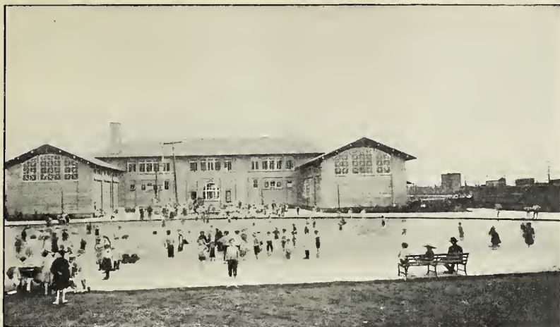
Courtesy City Parks Assn., Philadelphia. Hamilton Park, Chicago. This shows a Neighborhood Center building. The construction throughout is of concrete. The central part contains the assembly hall, refectory and clubrooms. Each wing contains a gymnasium with locker rooms and shower baths with plunge. One is exclusively for men, the other for women. The wading pool is of ample proportions, and nothing delights the youngster more than to splash around in it and sail toy boats.
